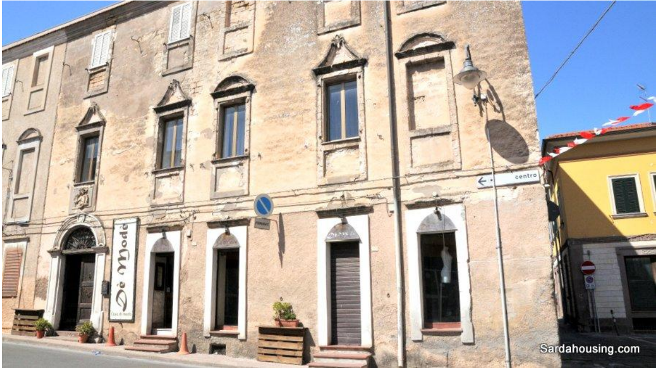
1 – Ittiri – Sassari: House Castello – Corso Vittorio Emanuele: front side of the building
