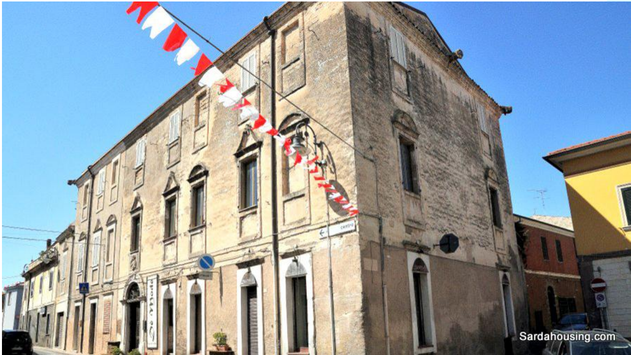
18 – Sassari: House Castello – Corso Vittorio Emanuele: the 18th century building
