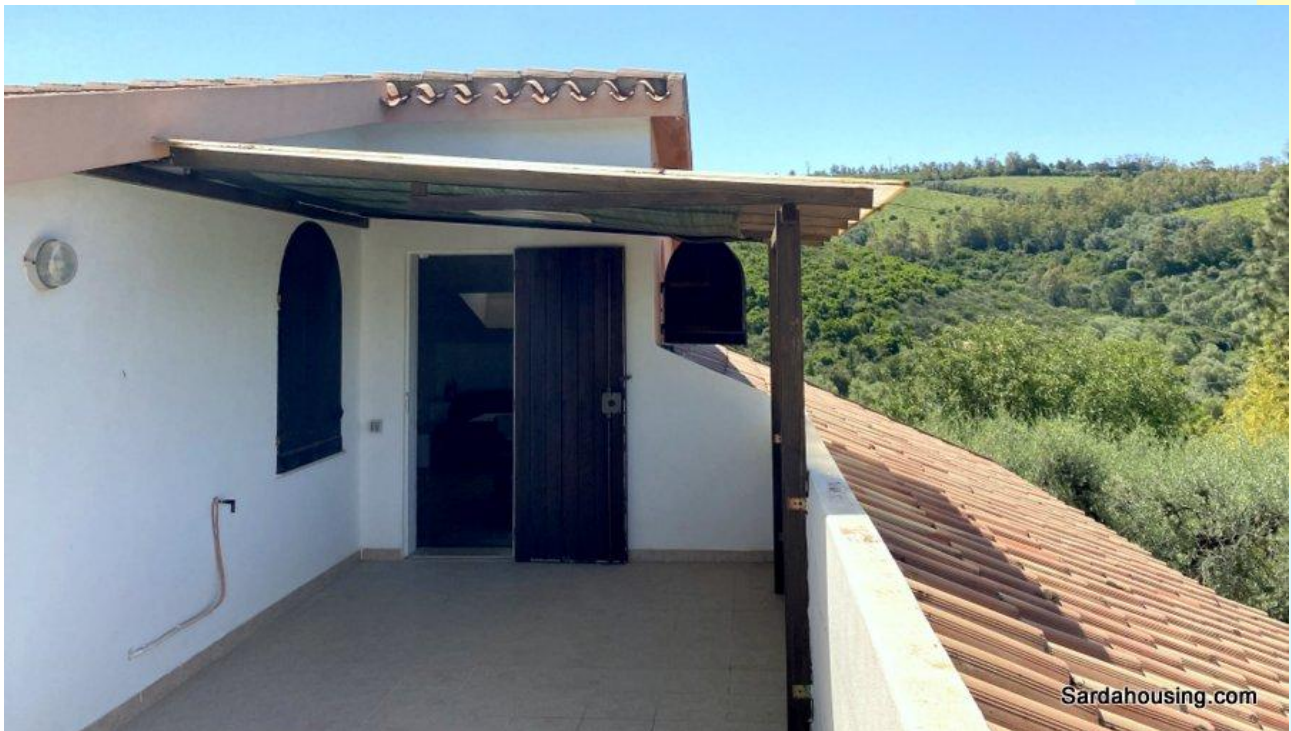
26 - Soleminis – Cagliari – Villa Cavana: terrace and attic entrance
