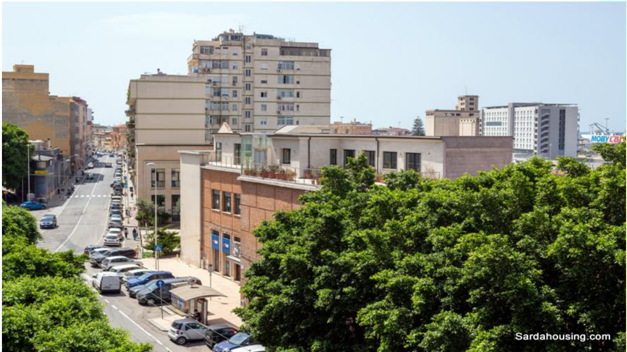
12 - Cagliari, viale Trieste – Apartment Trieste: a view from a balcony
