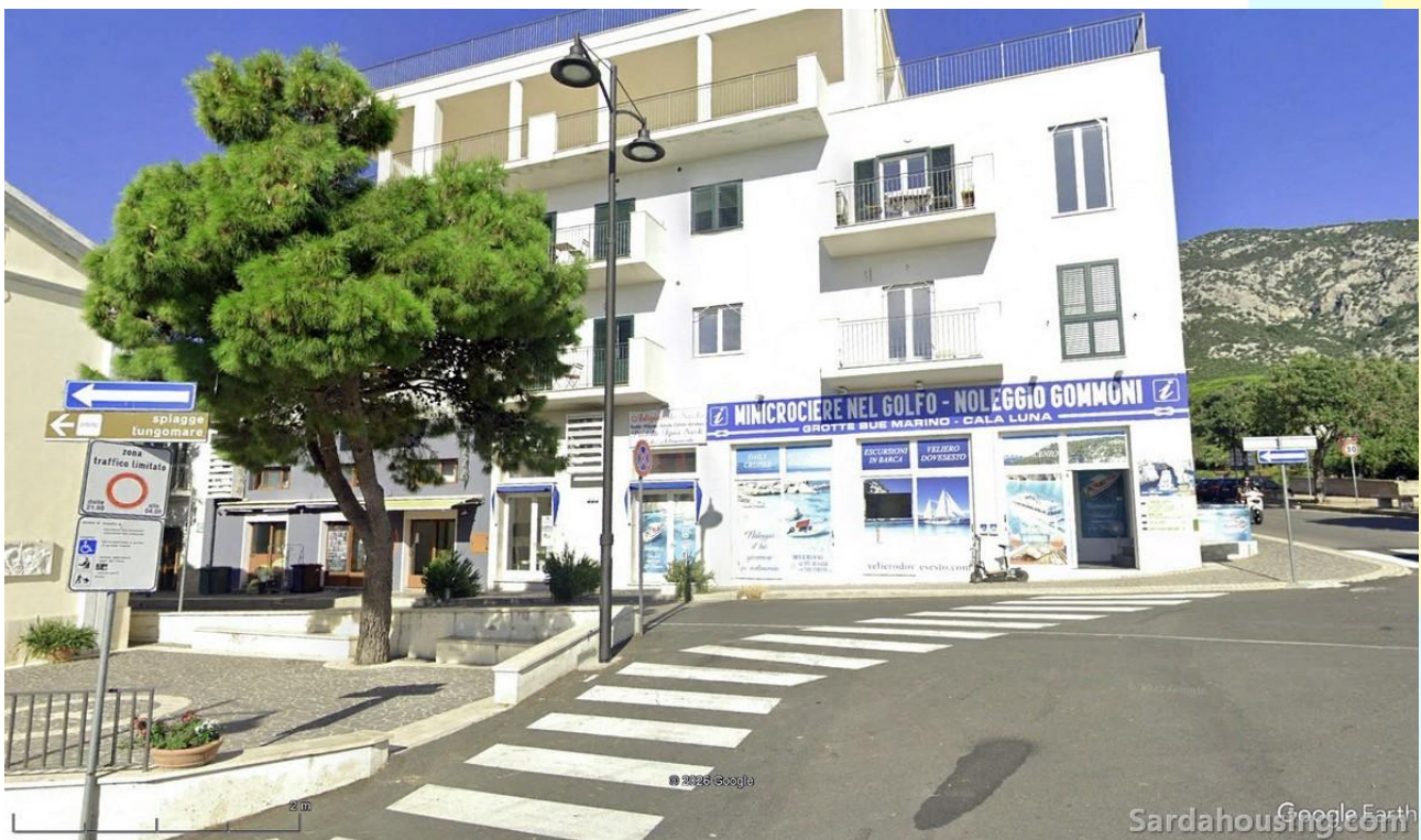
22 - Cala Gonone – Dorgali – Apartments Amerigo: completely renewed building
